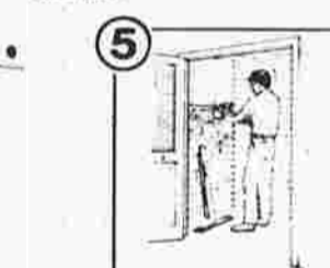
Finish back wall first, then do the side walls.
